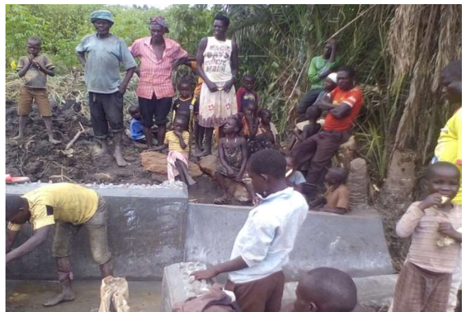
Completing a spring well Masindi District, Uganda
